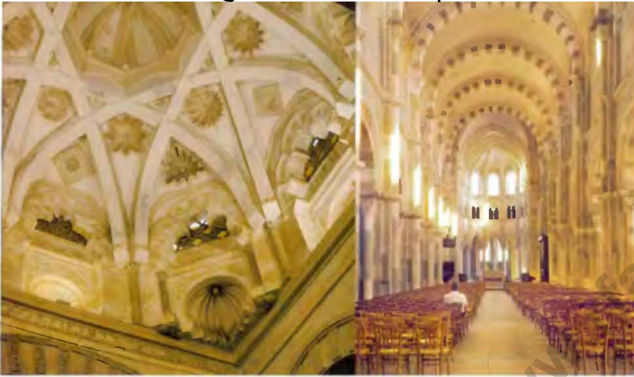
Left to right: Rib vaulting in the maqsura dome of the Great Mosque of Cordoba, added in the 10 th century; ribbed, tunnel vaults at 12 th -century Sainte-Madeleine in Vezelay, France, resembling those of Susa, built in 821–822.
