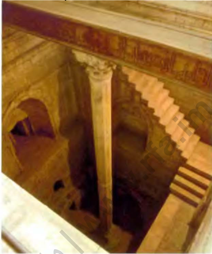
The nilometer in Rawada Island at Fustat, near Cairo, completed in 861-862 CE. The octagonal column in the centre is used to measure the height of the water in the Nile in cubits.
