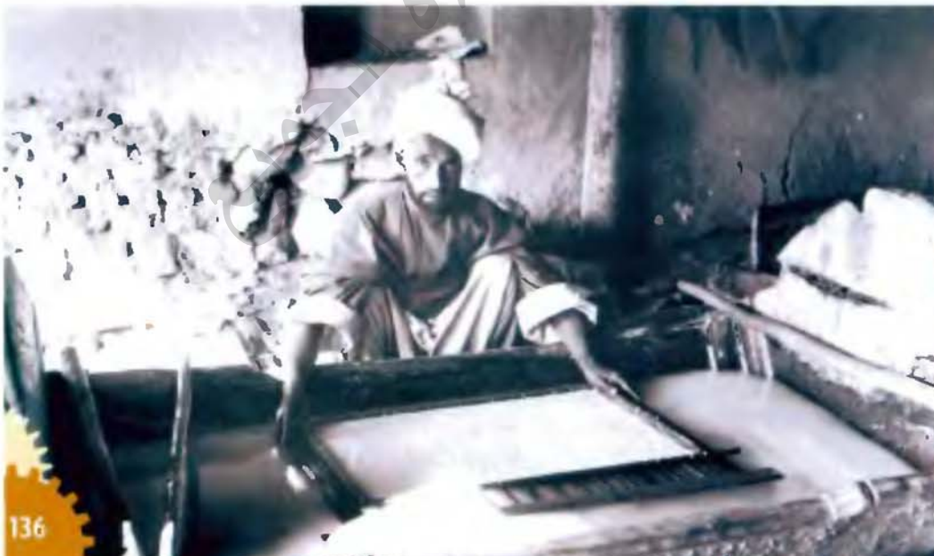
Left to right: Ancient methods of forming sheet paper can be seen here, as a vatman forms a sheet of paper in Kashmir, India, 1917; 17 th -century manuscript showing the papermaking process.
